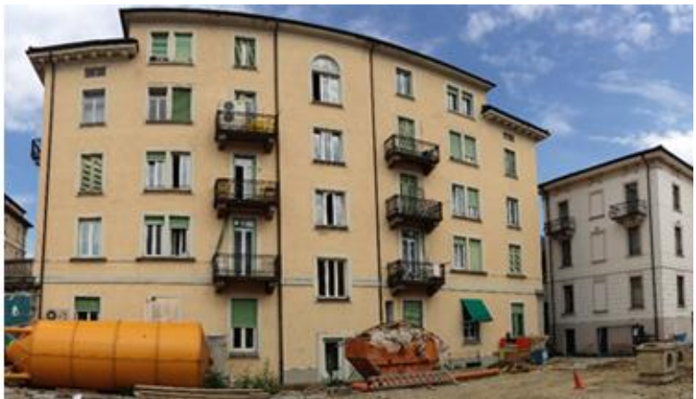
Fig. 1. Palace G. Guisan Street (A4907). East (a) and West (b) facades.
