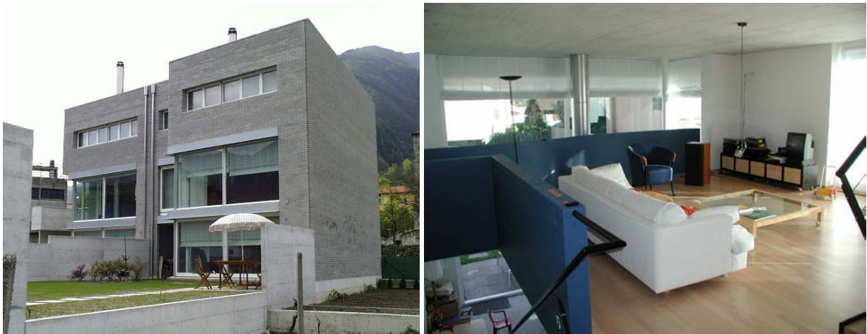
Figure 1: South-east façade and interior of the “Vitali-Velti” house.
