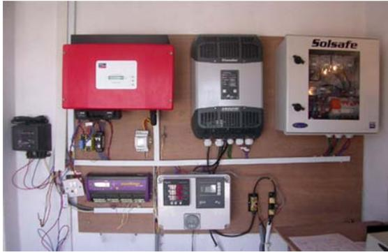
Figure 3: 1.1 kWp PV system with a back-up battery at the main head office of RIDS-Nepal in Imadol, Lalitpur district (P3).
