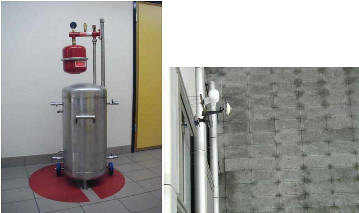
Figure 5: Buffer tank (left) and climatic data probes.
