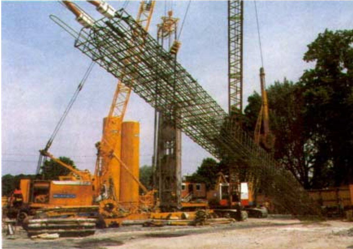
Fig. 1.4 Metallic reinforcement of a cast-in-place wall imbedded in the ground. The pipes for the heat transfer with the ground are fixed in the reinforcement (source: photo Nägelebau, A-Röthis).
