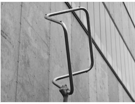
Fig. 12: The table trestle and the facade of the new building share the same surface coating.
