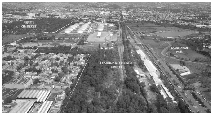
Fig. 4: 18 de Marzo Oil Refinery. Current conditions of the study area (308 acres). There is potential for developing a vision that sets an attitude at an urban scale. Photo credits: Stock Aereo, 2019. Diagram: Jorge Zapata.
